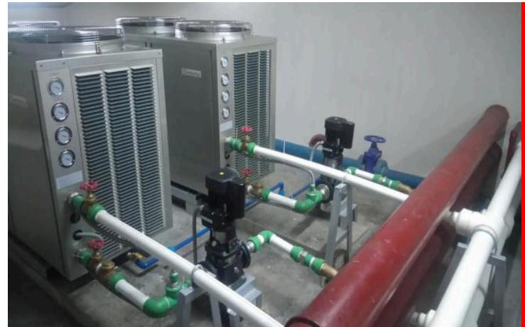
Rheem Air Source Heat Pumps gather ambient air and transfers the heat from the air into the water. Taking efficiency to the next level, Air Source Heat Pumps exhaust cold air in the process, and can be ducted back into the establishment as an additional source of intermittent air cooling.
